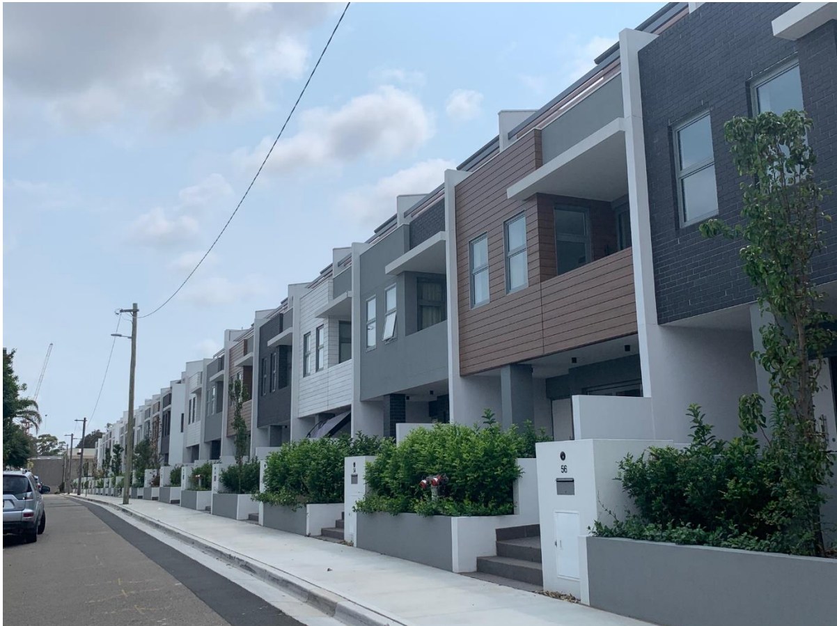
Figure 33: Salisbury Lane frontages of three-storey town house dwellings at 50-86 Dunning Avenue, Rosebery.
