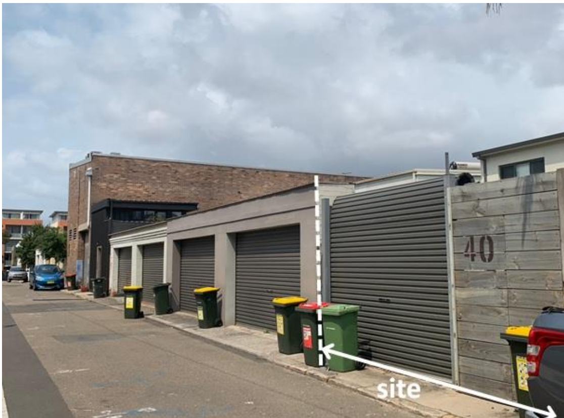
Figure 7: View south along Salisbury Lane.
