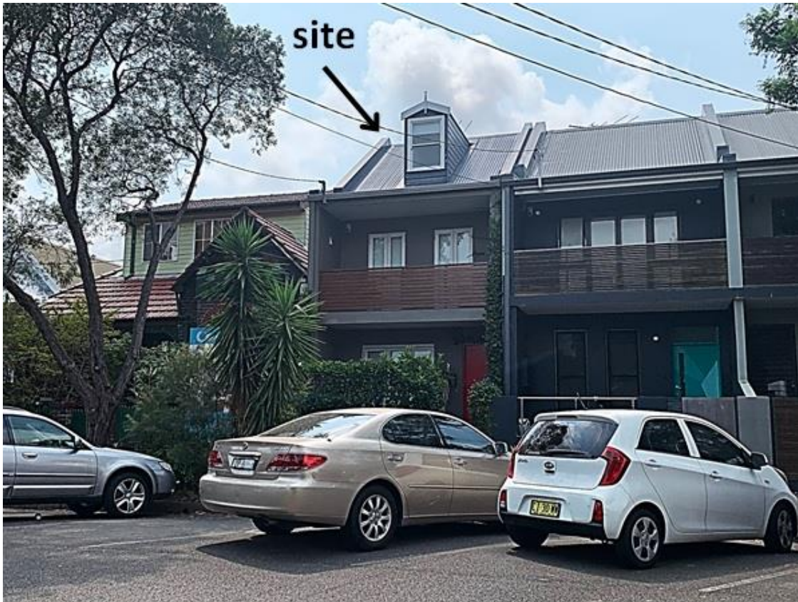
Figure 2: Site viewed from Princess Avenue.
