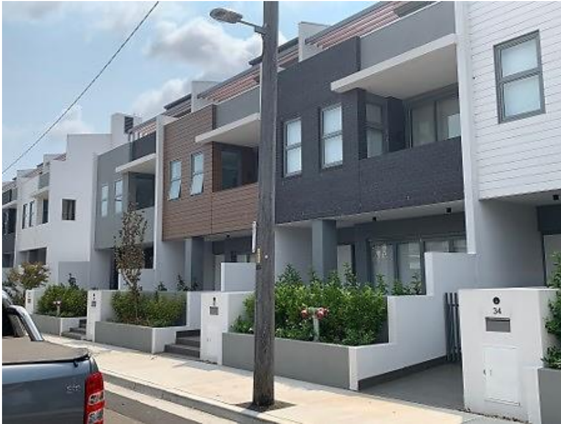
Figure 4: Salisbury Lane frontage of townhouse development at 50-86 Dunning Avenue.
